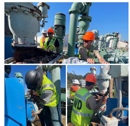
EMAC crews from Littleton, Massachusetts replace valves in conventional raw water pumps today at the O.B. Curtis water plant in Jackson. These valves ensure that the proper volume of water enters the treatment process.
