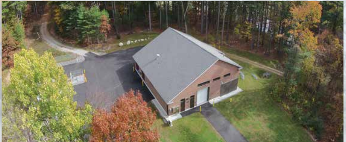
The Beaver Brook treatment plant is similar in size and design to the proposed Whitcomb Ave. facility.
