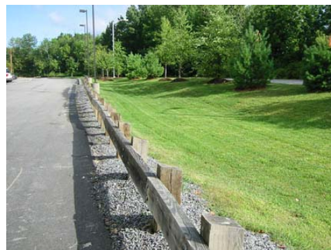
This dry swale absorbs runoff from the adjacent hotel parking lot.
