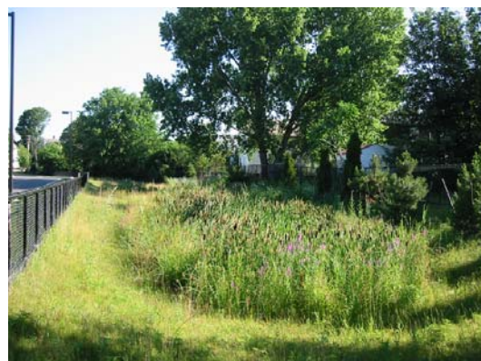
This stormwater wetland has a healthy cattail population and treats stormwater at the McGlynn School in Medford, Massachusetts.
